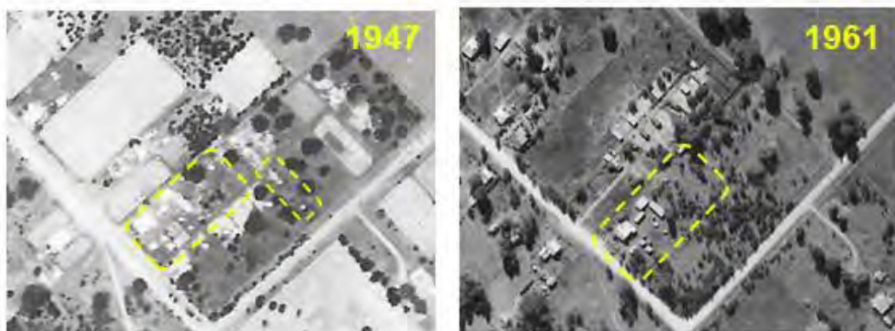
Figure 1: C.1890s stone cottage complex with various outbuildings and structures indicated on historical aerials
